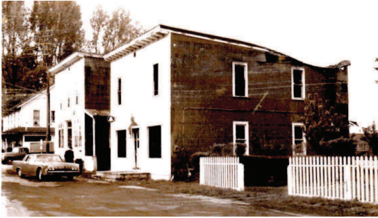
Brant Center Fire Damaged Buildings May 14, 1964 Joseph Iripi, owner
